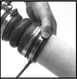
Evenly space the two hose clamps over the stern tube end of the hose. Stagger hose clamp drives on either side of the hose to distribute pressure evenly. Make certain the drives are accessible. Confirm that hose clamps fully engage the SureSeal™ and the stern tube. Tighten clamps.
